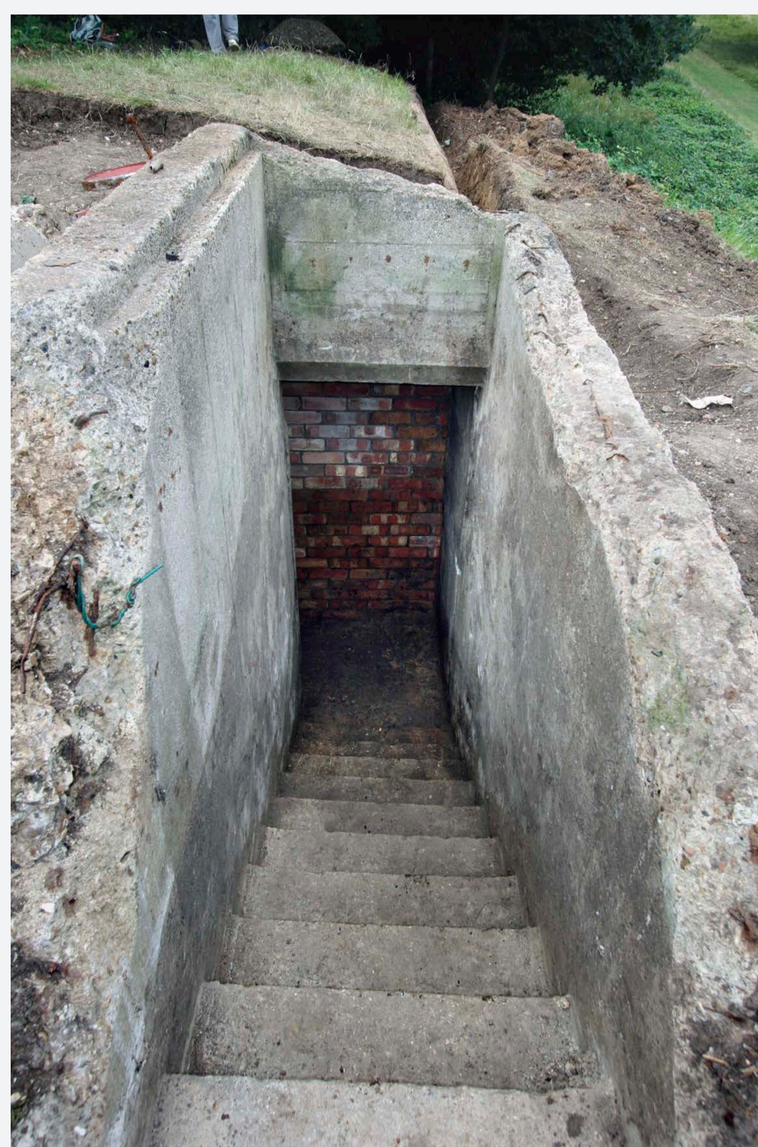
Figure 5: the staircase entrance following excavation. Photo G. Moshenska
