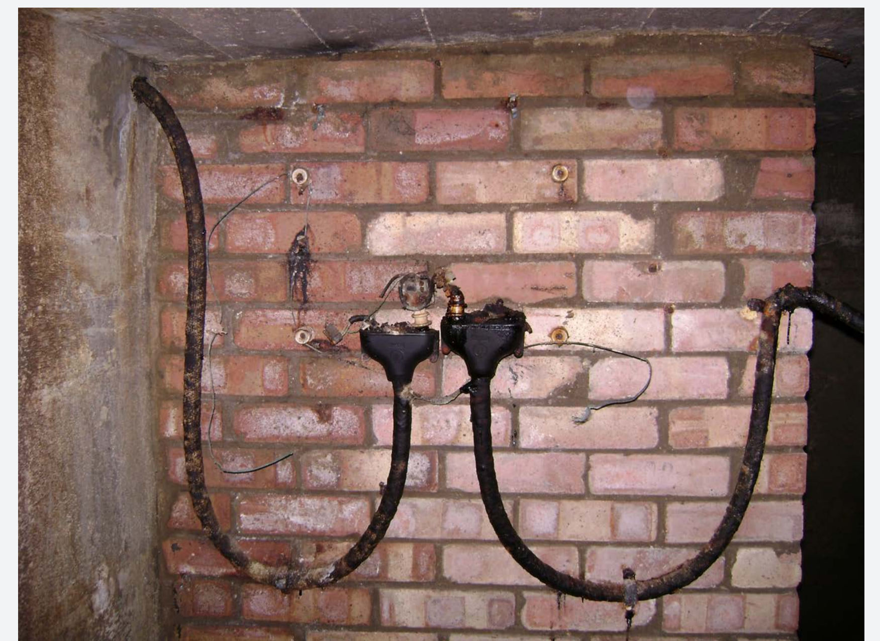
Figure 6: electrical fittings inside the shelter. Photo G. Moshenska
