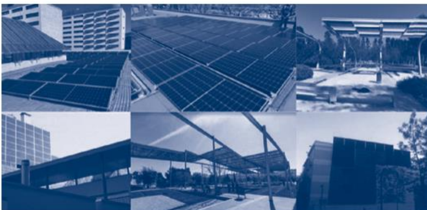
Image 1. Photovoltaic installations on municipal buildings
