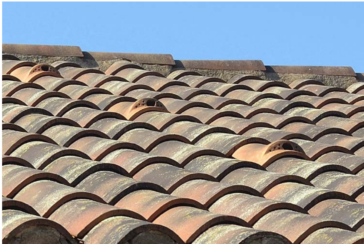
Roof tiles for swallow nesting
