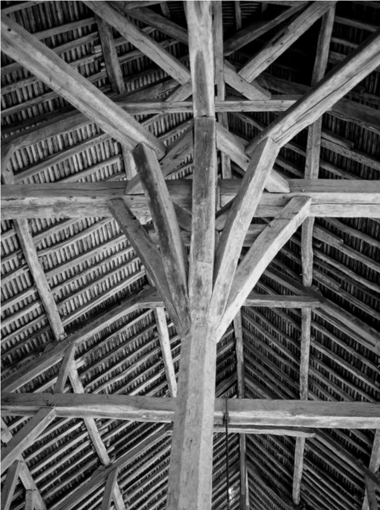
Mediaeval market in Mereville. Detail of the structure
