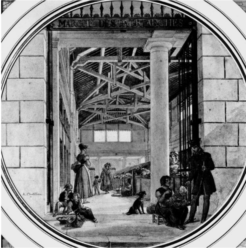
Marché des Patriarches, 1828-1831. Architect: André Chatillon. The wooden framework closely resembles those of market halls built at the end of the Napoleonic Empire
