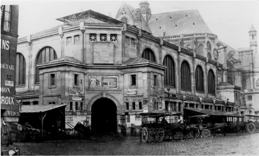
The first stone pavilion, completed in 1854. Its volume, narrow openings and solid, closed appearance won it the name Fort de la Halle among Parisians, despite the fact that the interior was covered by a cast-iron structure. It was eventually replaced by pavilions made entirely of cast iron
