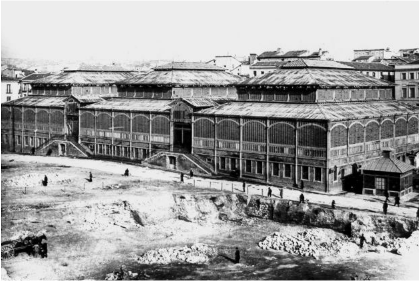
General view of Los Mostenses Market, no longer extant, Madrid, 1867-1875. Architect: Mariano Calvo Pereira
