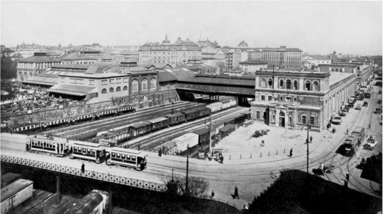
The new meat market, 1898-1899, in front of the Viktualienhalle, 1904-1906. Connecting bridge to the wholesale market
