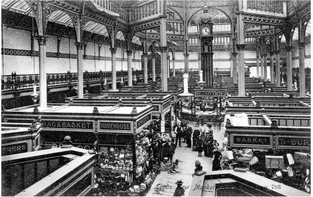
Kirkgate Market Hall, Leeds, 1904. Architect: Leeming and Leeming
