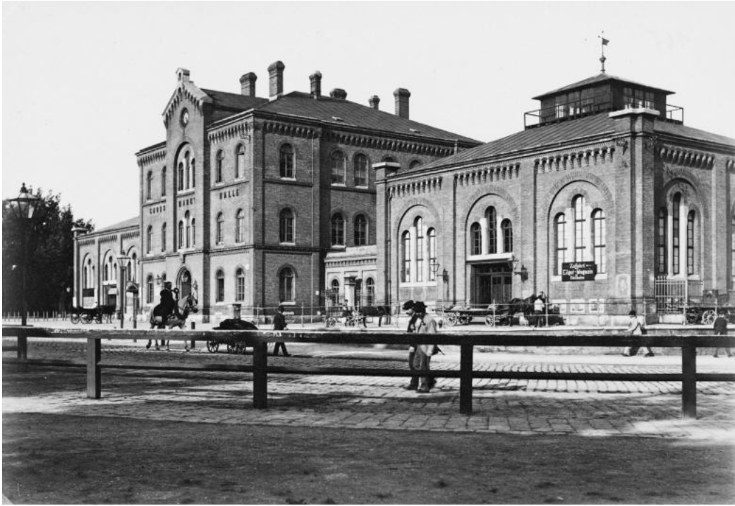
Exterior view of the Zentral-Markthalle. Karl Gabriel and Georg Haussmann
