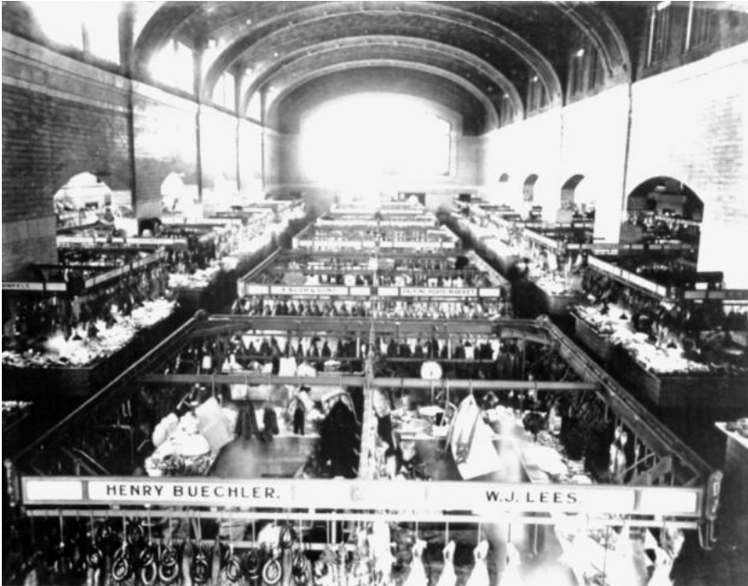
View of the interior of West Side Market, Cleveland, showing the vaulting made by the Gustavino Company, 1912
