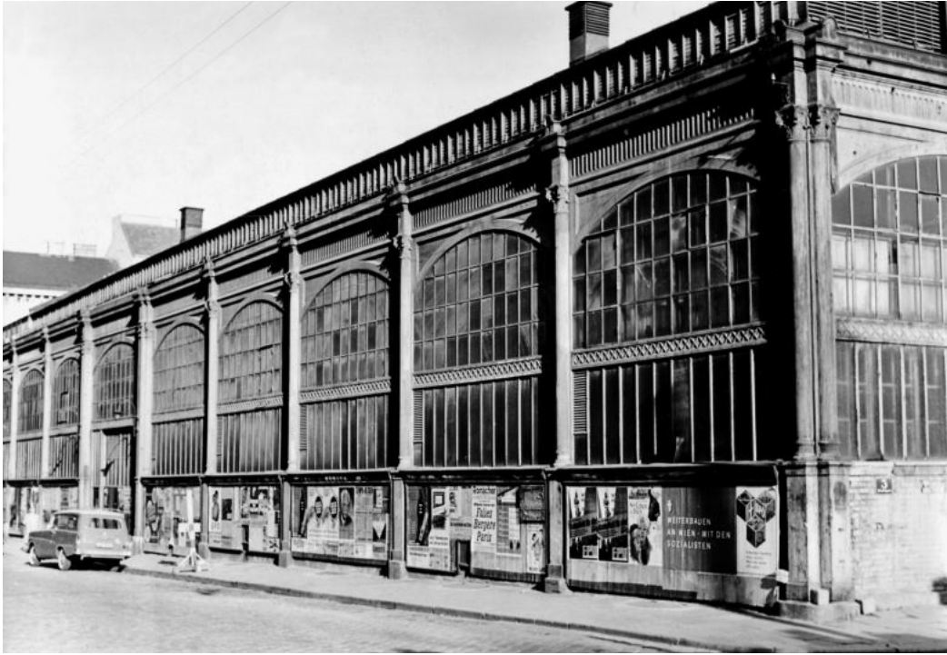
Exterior view of Zedlitz Market, 1869-1871. Architect: Georg Haussmann
