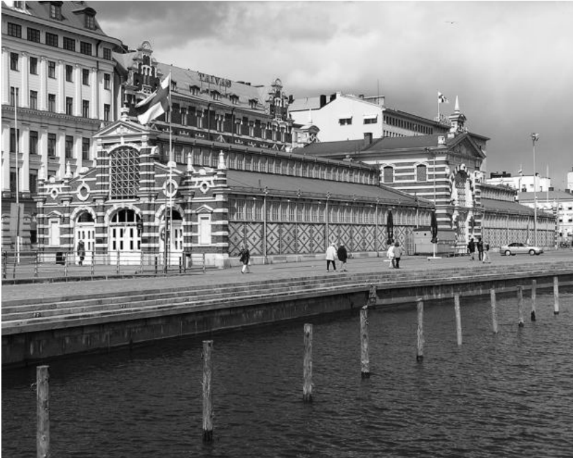
Wanha Market, Helsinki, 1889. Architect: Gustaf Nyström
