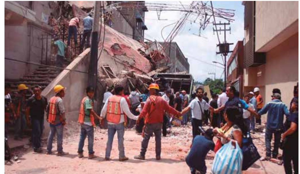
Earthquake damages in Mexico (September 2017)
